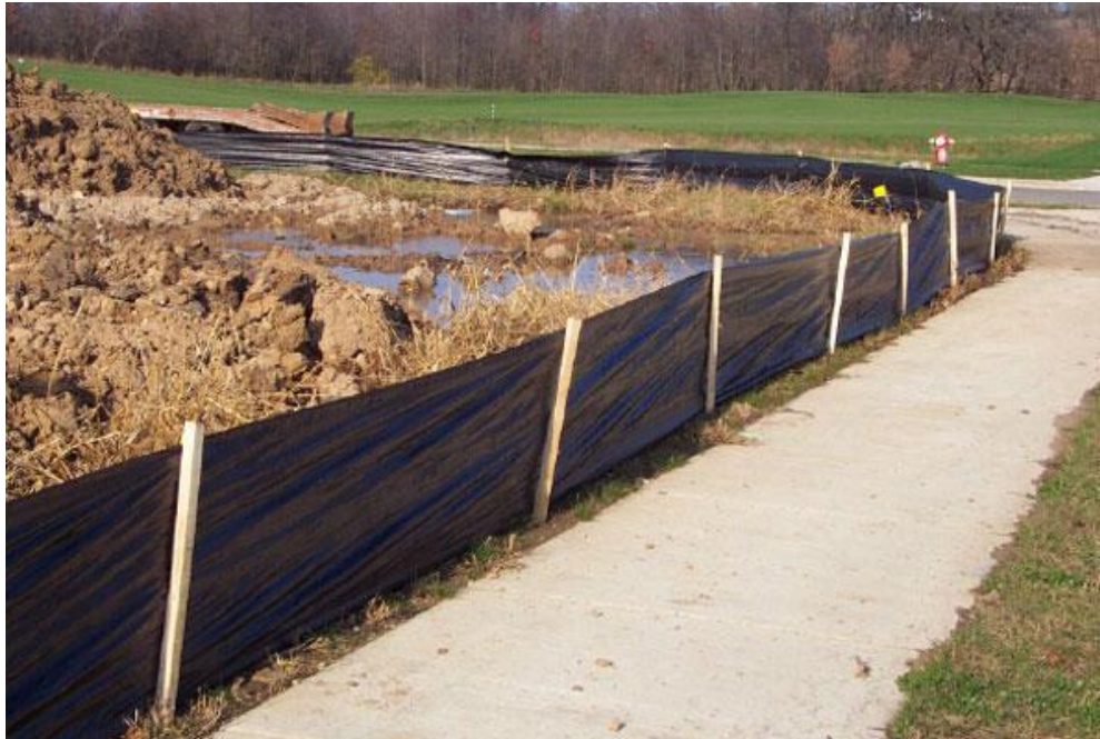
Figure 6.2 Typical Silt Fence to be Employed
